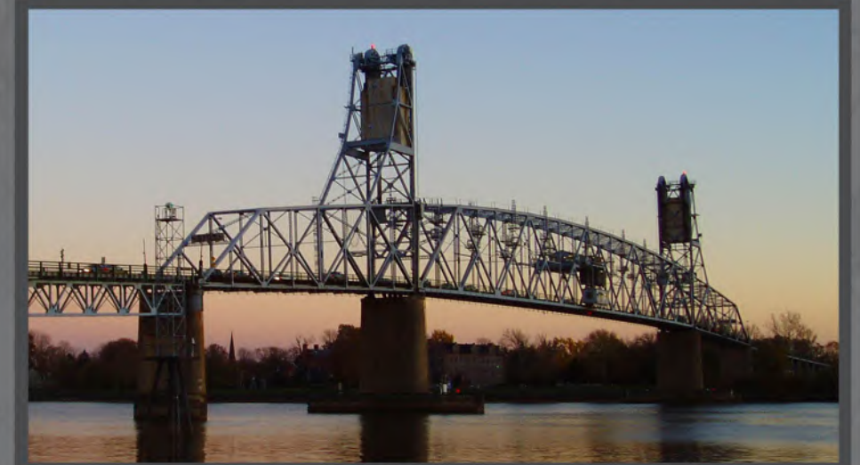
BURLINGTON BRISTOL BRIDGE
